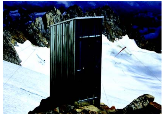
Construction of the new outhouse. Photos - D. Hughes.
