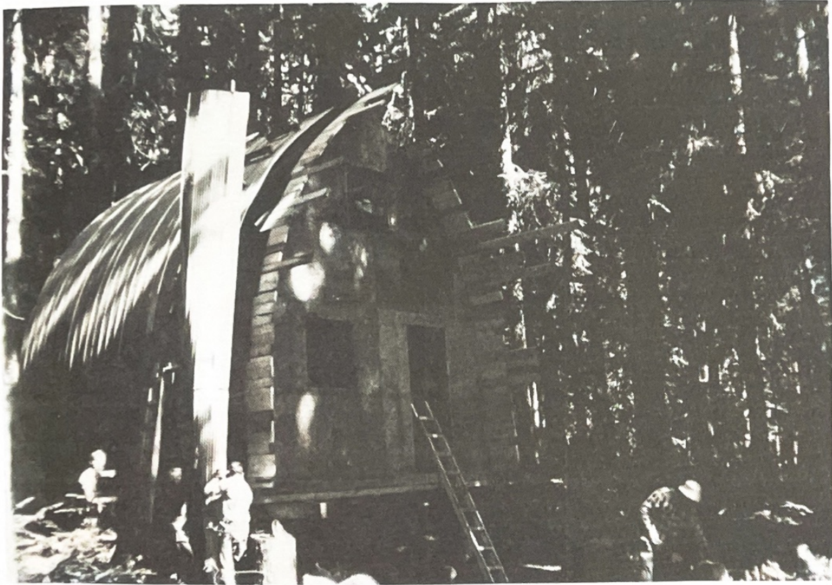
The roof is almost on. Photo - P. Crean.
