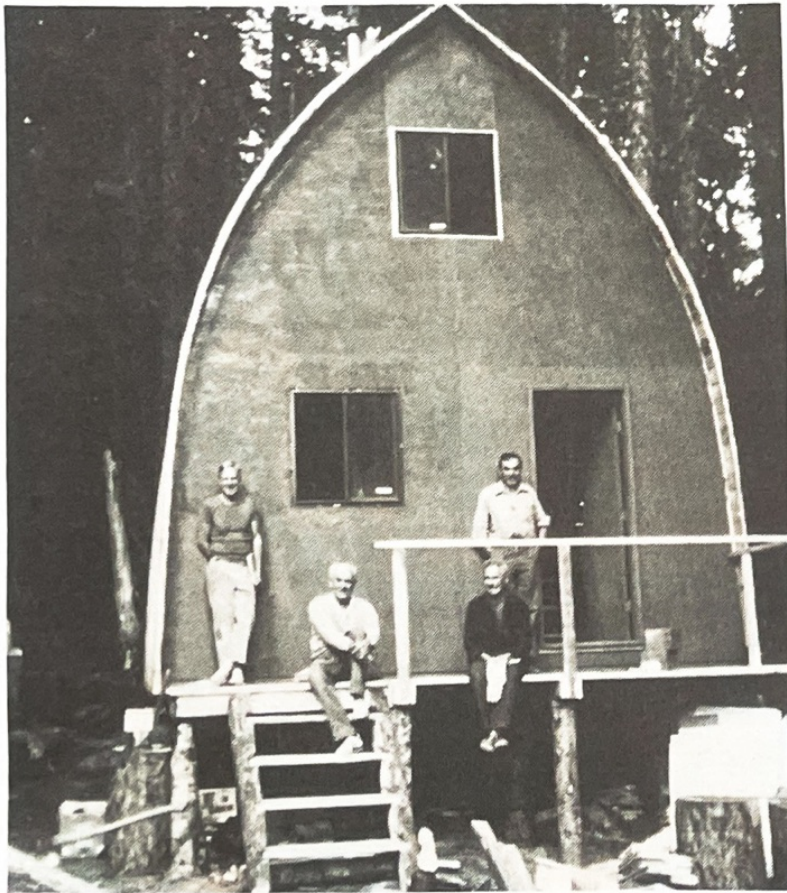
Some of the cabin builders (from left to right - George Hamilton, Jack Apps, Howard Rode, and Pat Crean) relax after finishing the exterior. Photo - W. Saunders.
