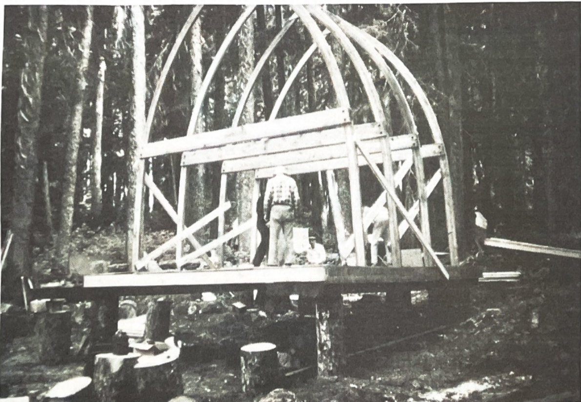
The cabin frame goes up. Photo - P. Crean.
