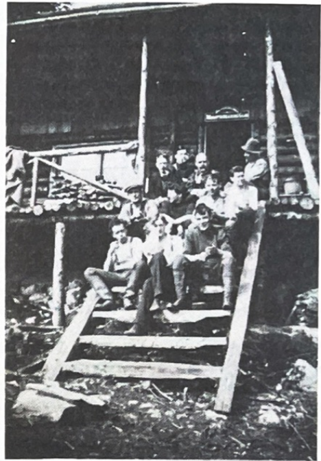
Construction of the first club cabin on Grouse mountain in 1910, and the cabin builders.
