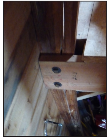
Split arches in the North Creek cabin caused by excessive snow load were recently repaired. Photos: Emanuele Porra
