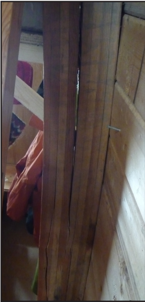
Split arches in the North Creek cabin caused by excessive snow load were recently repaired. Photos: Emanuele Porra
