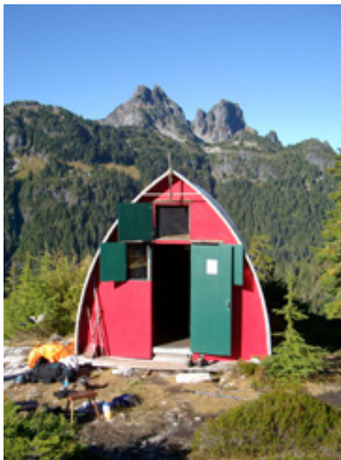
Rejuvenated Mountain Lake cabin. Photos - Julia Borchardt.
